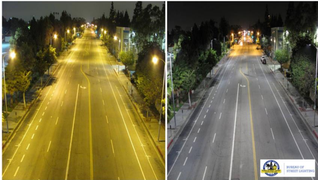
Figure 8 - Replacing HPS streetlights, which have poor color rendering and higher energy costs, with LEDs has a significant impact. For example, LED implementation has resulted in 64% energy savings for the City of Los Angeles, while still meeting the LABSL standard of 3000 K and > 70 CRI for LED installations. Photo credit.
